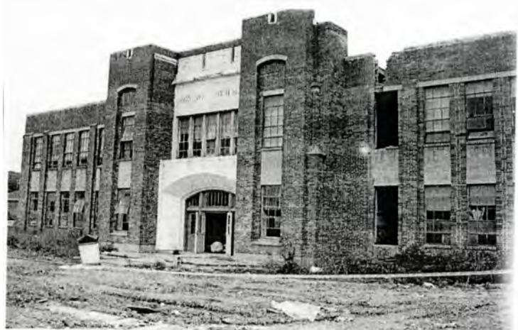
Huntsville High being demolished and rebuilt in 1994
