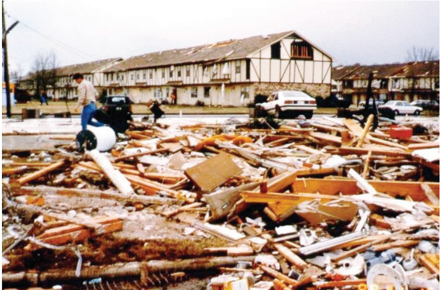
Waterford Square Apartment Damage
