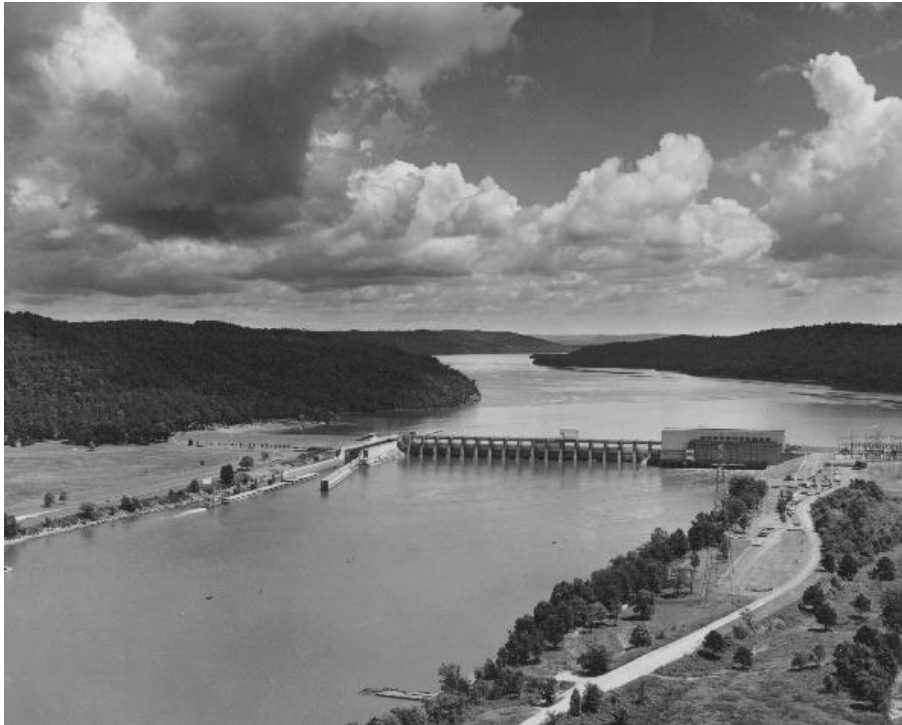
View of Guntersville Dam from the south side of the Tennessee River.
