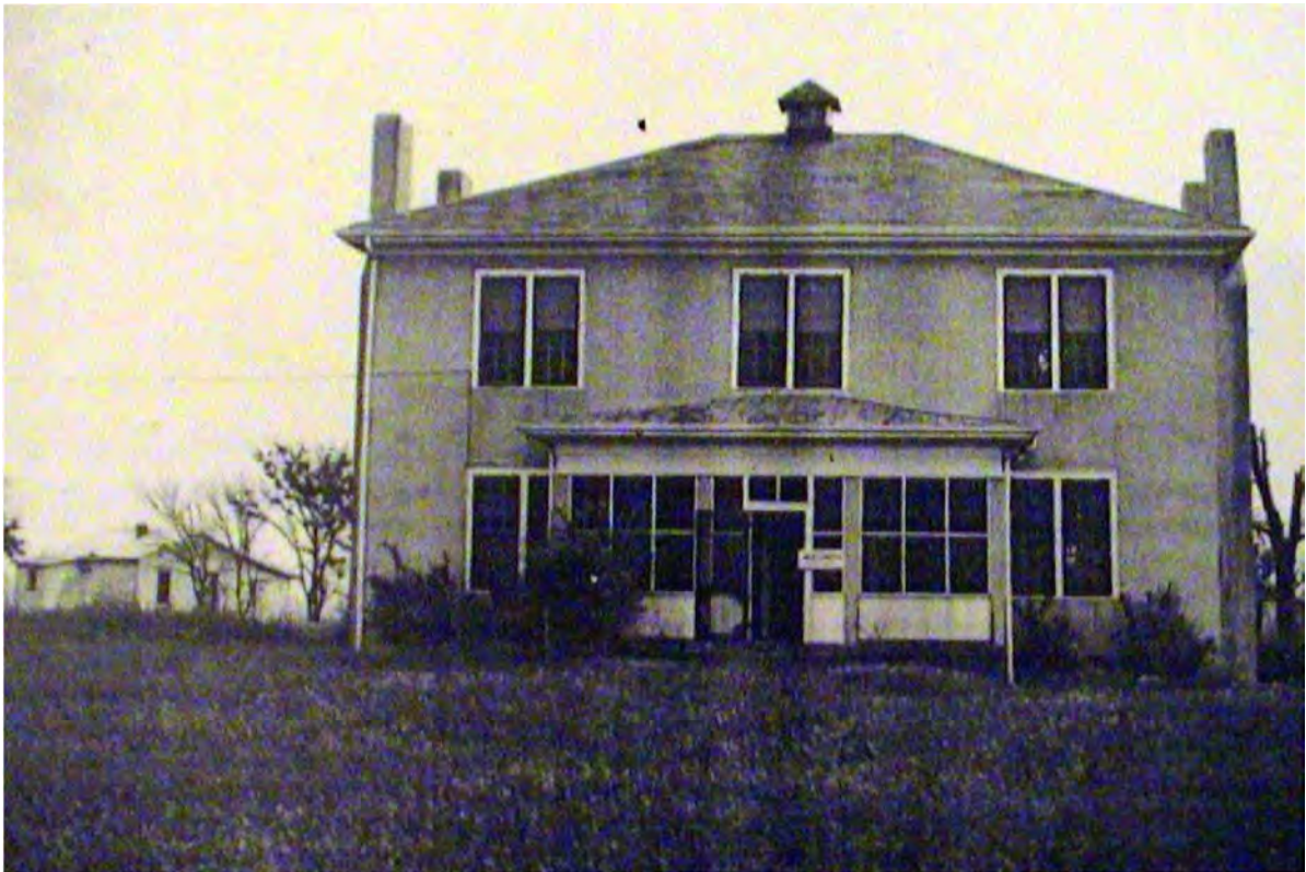
The Chaney House on Parcel A-17 had a stucco exterior and a chimney on each corner. Notice the structure behind the house to the left. Source: The Redstone Rocket , October 25, 1989, p. 10.
