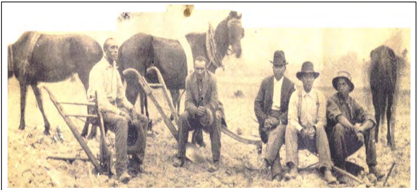
Groundbreaking day for the Horton School. The men pictured were the trustees of the school. They were: Frank Jacobs, Henry Lacy, Wattie Timmons, Yancy Horton, and Alva Jacobs. Yancy Horton donated the land for the school; he and the people of the Pond Beat community built it. [Alva Jacobs who is pictured was the uncle of the boy of the same name who is in the story presented above.] NOTE: According to the source of this photograph, Pearl Horton Higgenbotham, when the photograph was published in the July 2, 1980 edition of the Redstone Rocket , the men were identified incorrectly, thus, they may be identified incorrectly in other places where the photograph is on record.
