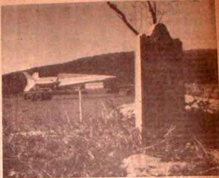
UNDISTURBED — Just a few yards off Patton Road — the main thoroughfare at Redstone Arsenal—is a cemetery. A Nike-Hercules anti-missile missile passing the cemetery illustrates the change which has taken place at the government installation since the person whose grave is marked by this tombstone was buried. However, despite the drastic switch of the area from a quiet country place into use of the busiest places in the country, this graveyard and about 59 others on the Arsenal property have not been molested and are, in fact, kept up by the Army. (Photo by L.L. Cecil Staughton)
