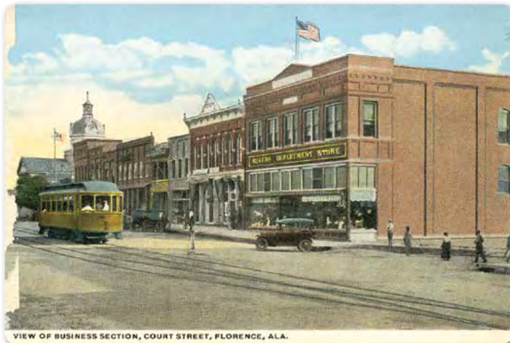
VIEW OF BUSINESS SECTION, COURT STREET, FLORENCE, ALA.
