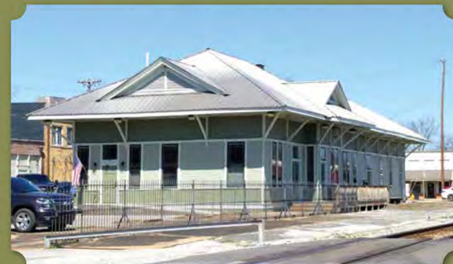
(Left) Restored Window inside the Athens Depot-Limestone County Archives, Athens, Alabama (Photograph by Jenna Tran) (Below) Athens Depot-Limestone County Archives, Athens, Alabama (Photograph by Jenna Tran)
