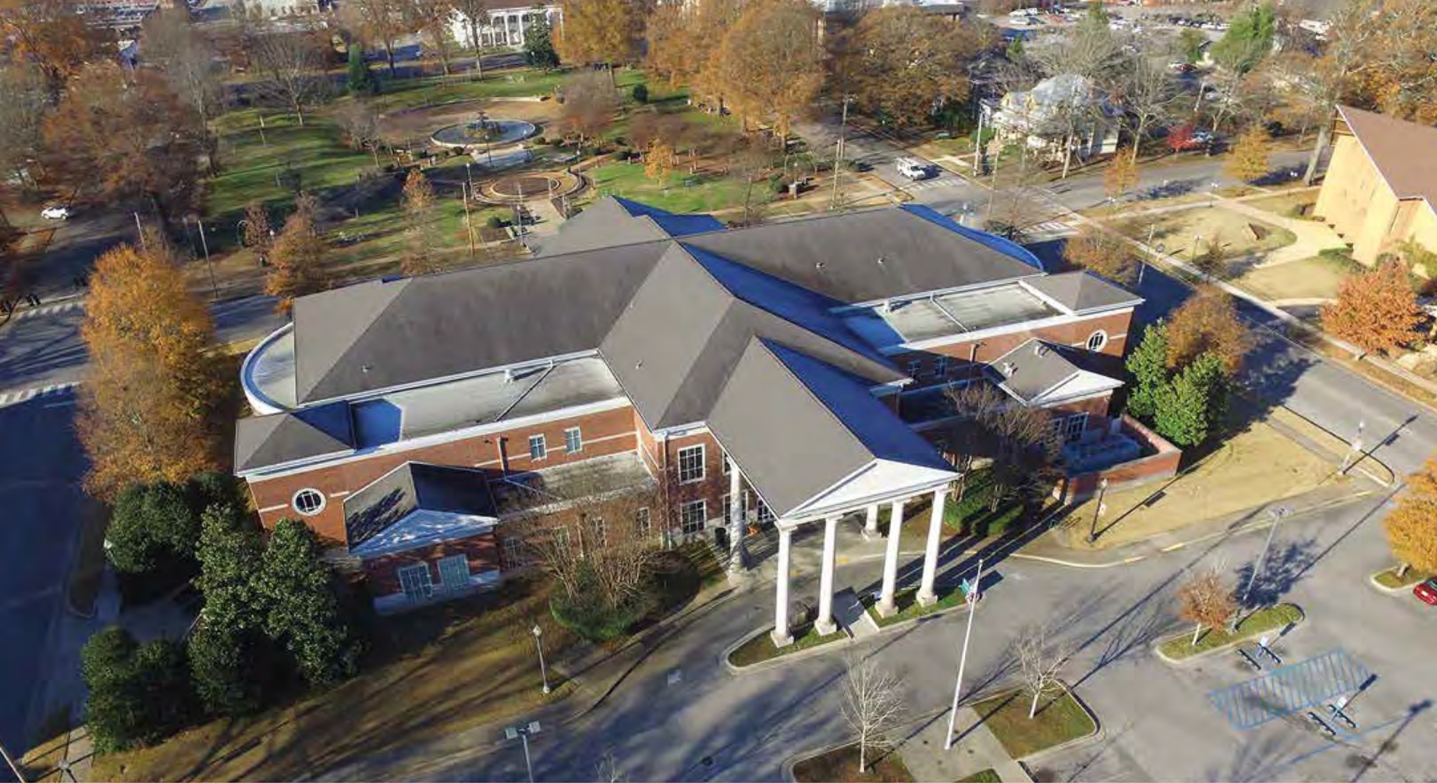
(Above) An Aerial View of the New Florence-Lauderdale Public Library from the East with Wilson Park and the Regions Bank (Forks of Cypress Look-a-Like) in the Background (Florence-Lauderdale Public Library)
