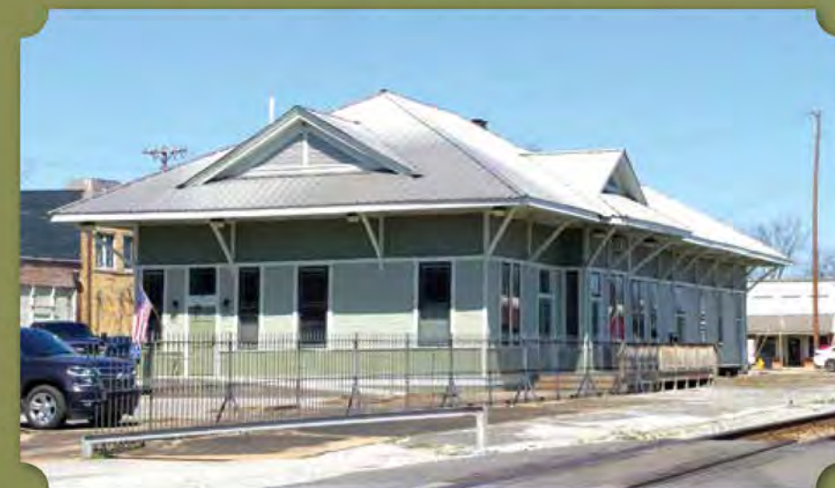
(Left) Restored Window inside the Athens Depot-Limestone County Archives, Athens, Alabama (Photograph by Jenna Tran) (Below) Athens Depot-Limestone County Archives, Athens, Alabama (Photograph by Jenna Tran)
