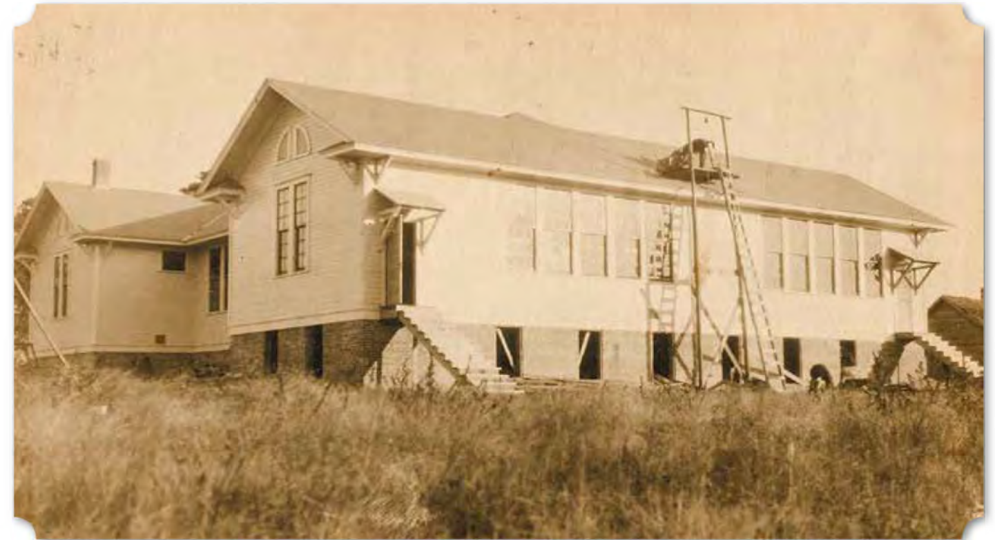
(Above) Morgan County Training School Being Built 1924 (Fisk Rosenwald Database)
